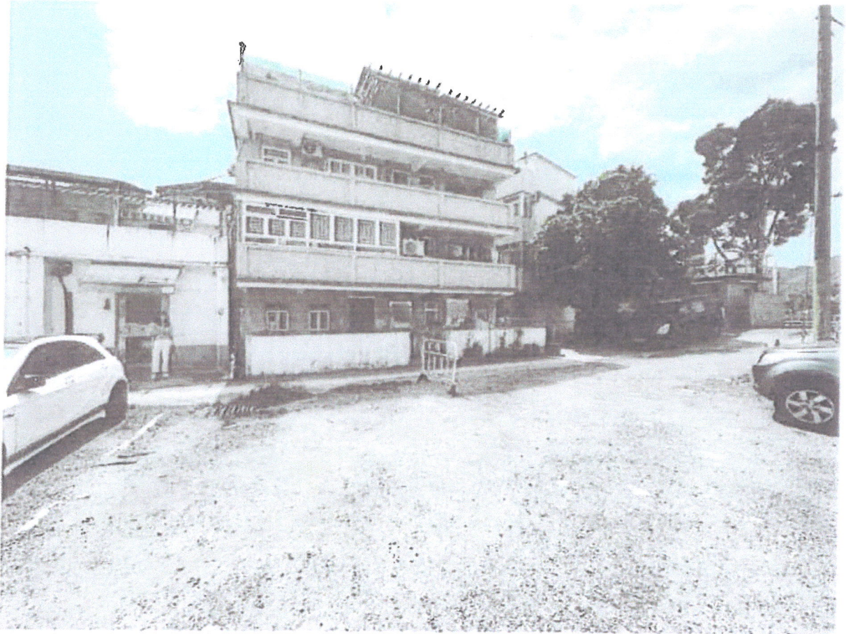
PHOTO NO. 5 Conditions of the Site
